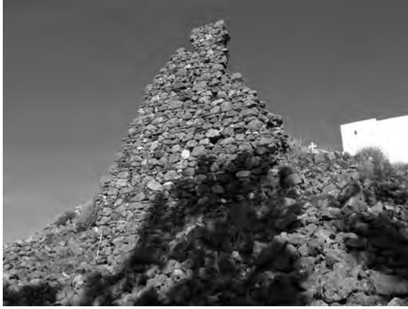
Fig. 6.43 View of tower 6 from the South
