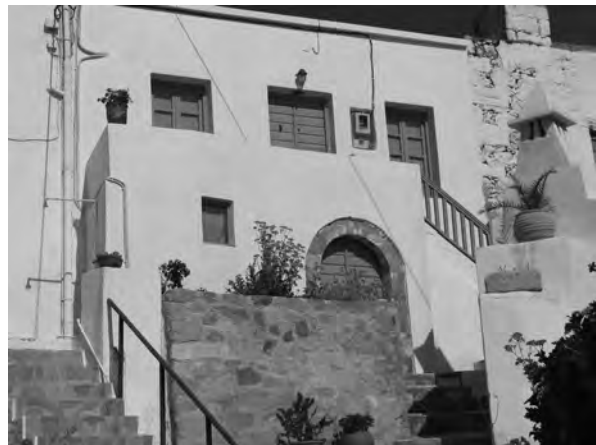
Fig. 6.70 View of a broad-fronted two-storey house in Plaka, Melos
