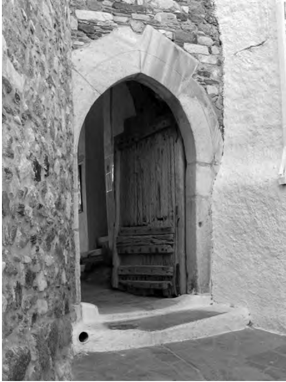
Fig. 5.27 View of Trani Porta , the main gate of Kastro on Naxos
