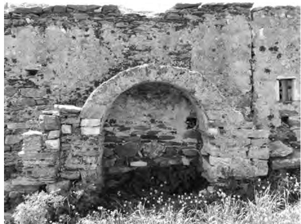
Fig. 6.123 Arch-shaped structure built against the Northern wall of the church in area 37
