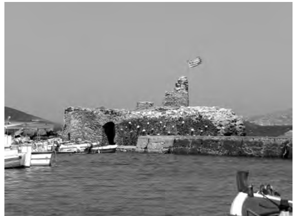
Fig. 5.9 View of the circular fort at the entrance of the Late Medieval harbour of Naoussa, Paros
