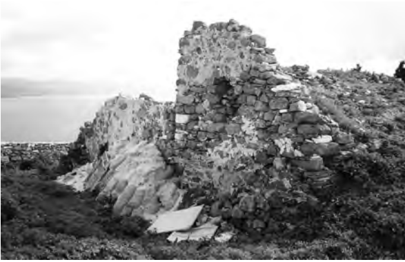
Fig. 6.41 View of the cistern and tower 5 from the Northwest
