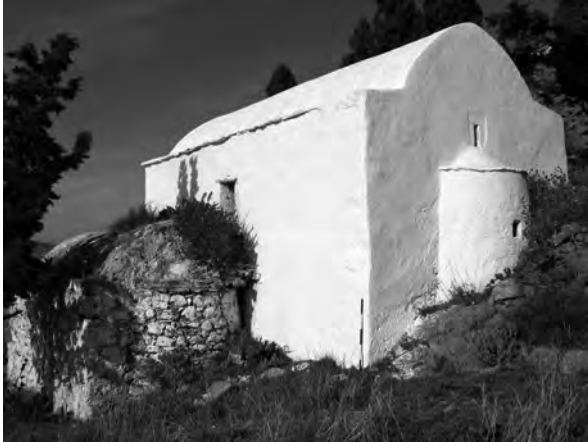
Fig. 6.37 View of chapels I and II from the Southeast
