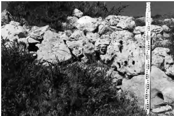
Fig. 6.4 View of the external facade of the defence wall on the Southeast side
