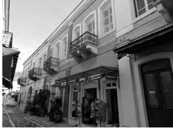
Fig. 5.24 Neoclassical houses along the main market-street of Paroikia, Paros
