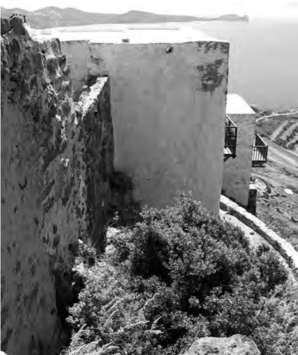
Fig. 6.57 View of the Northern defensive wall formed by the back walls of houses in the lower portion of Kastro on Melos
