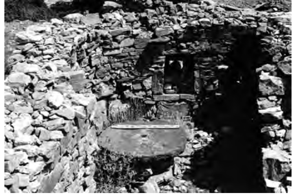
Fig. 6.88 View of the Eastern part of the olive-press building at Mavro Chorio
