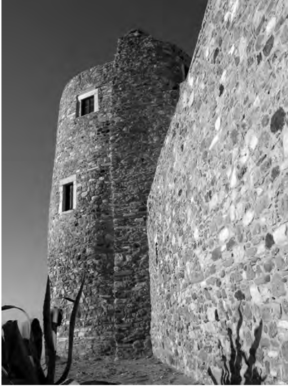
Fig. 5.15 View of the circular Glezos tower in Kastro, Naxos
