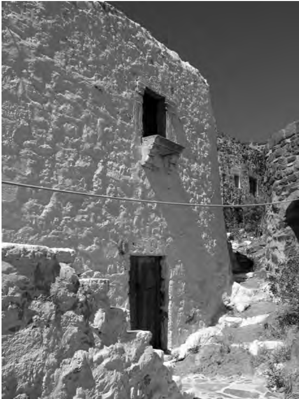
Fig. 6.61 View of a two-storey house in Kastro, Melos
