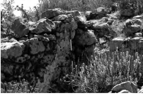
Fig. 6.48 Ruins of a house in area B with vaulted ground floor
