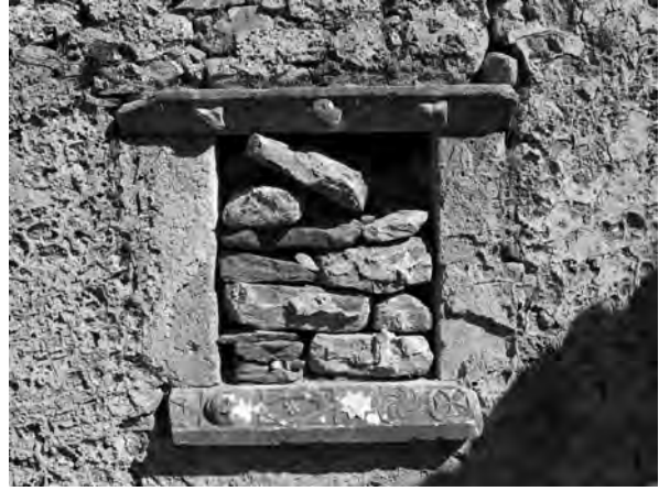
Fig. 6.18 Marble spolia from a Middle Byzantine church templon , used as window frames on the North wall of chapel 2 at Apano Kastro
