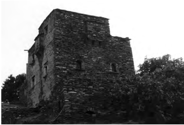
Fig. 5.54 View of the tower-house of Mastro-Yannoulis in Amolochos, Andros
