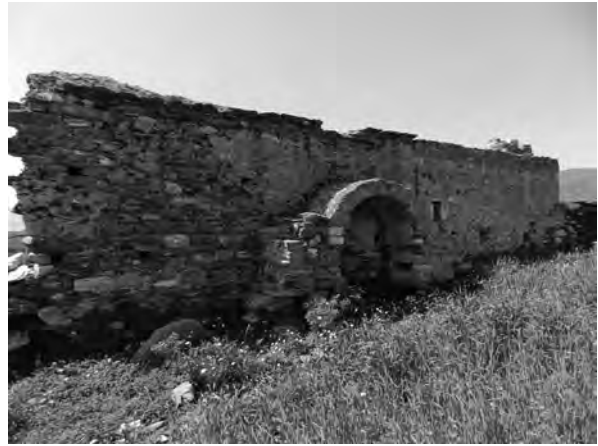
Fig. 6.122 View of the ruined church in area 37 from the Northeast
