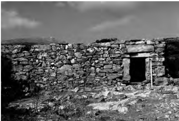
Fig. 6.92 View of house VI at Mavro Chorio
