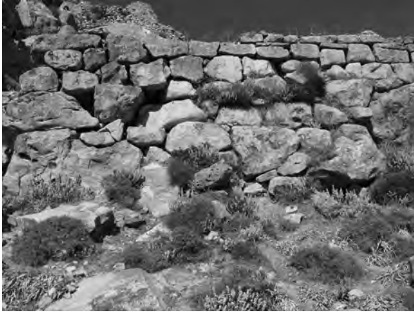
Fig. 6.14 View of the surviving archaic wall
