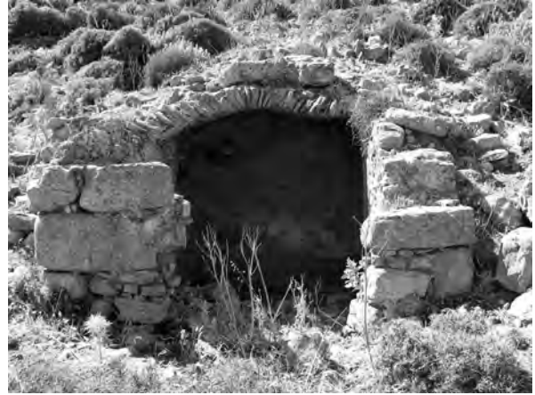
Fig. 6.21 View of cistern 3 at Apano Kastro
