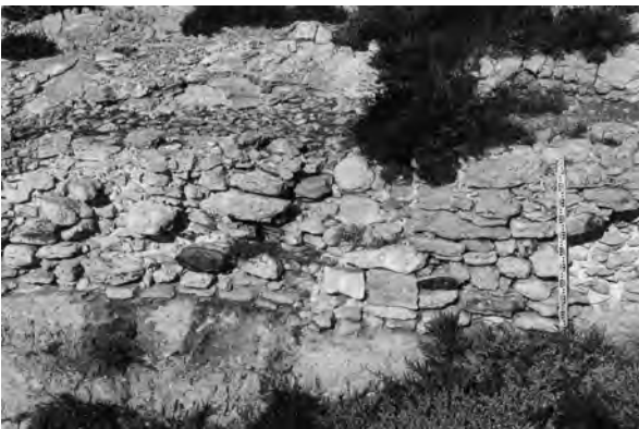
Fig. 6.8 Close view of the Northwest long wall of the sub-surface structure
