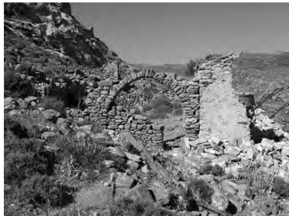
Fig. 6.26 View of the Southwest side of Hall B next to chapel II
