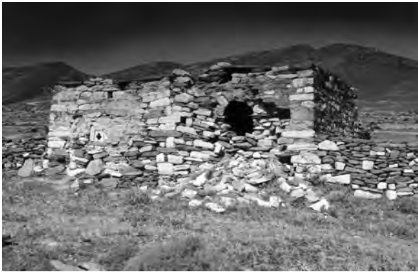
Fig. 6.125 View of the ruined twin-church in area 40 from the East
