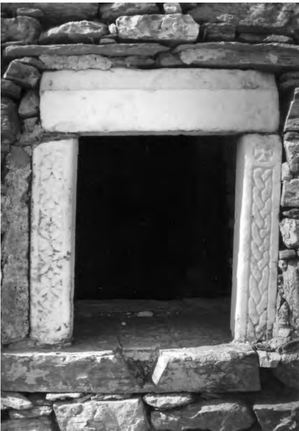
Fig. 6.128 Middle Byzantine spolia used as window-frames on the Northern wall of the twin-church on site 43
